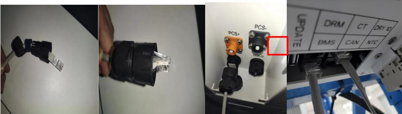
4. The ammeter connected to the three-phase circuit of the inverter, the ammeter and its communication line as well as the communication transfer interface belong to the inverter accessories, three CT ammeters respectively through three A\B\C three-phase (live operation is strictly prohibited), please note that the arrow direction on the ammeter should point to the direction of the inverter.
