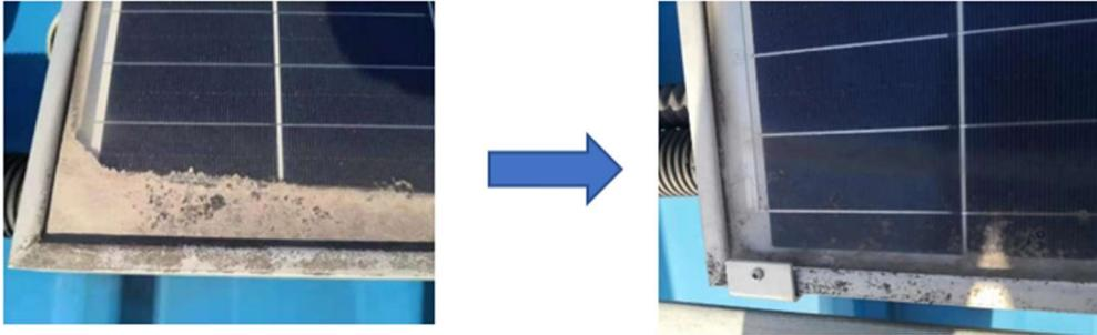
Such Mud builds up on the modules as the remaining water evaporates after a rain, especially if the modules are tilted below 15 degrees. Even if the modules are cleaned frequently, such mud triangle/strip will still grow up between cleanings.
