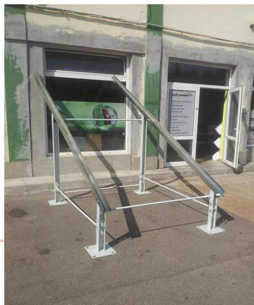
The frame (including modules) can be assembled in the composite without the anchoring. This allows you to precisely align the "finished" PV table.
