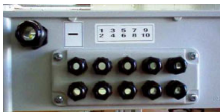
Figure 9-20: Cable gland for negative strings connection
